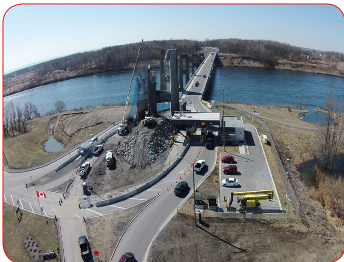
Aerial view of the toll plaza and the North Channel Bridge
