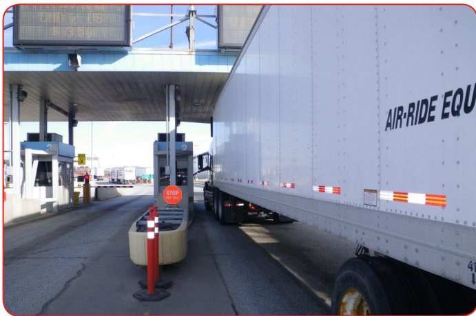
Toll booths at the Blue Water Bridge
