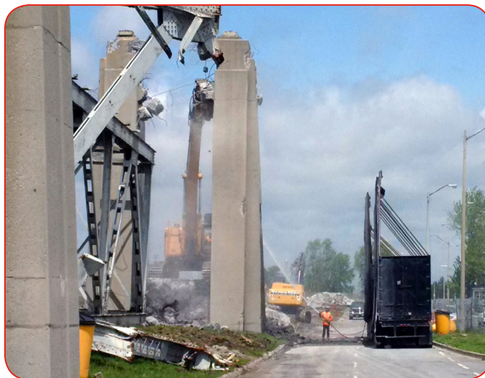
Pier demolition/steel structure removal in Cornwall
